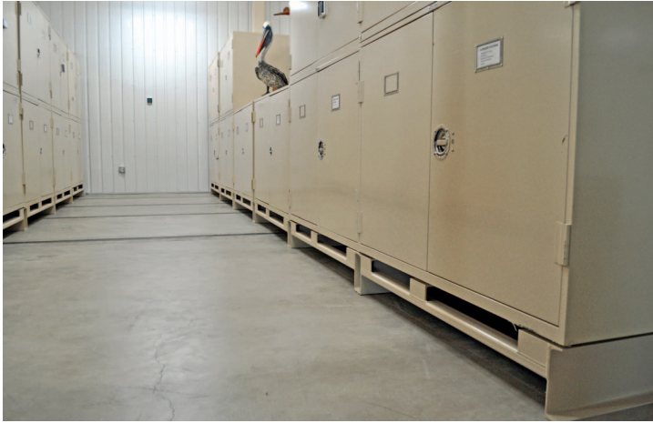
Figure 10. Cabinets with bird specimens raised 8 in. off the floor on custom-fabricated metal risers, February 2021.
